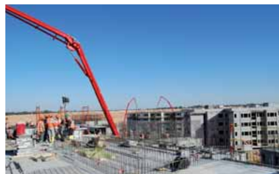
Concreting for our major customer Ranhill. Concrete work is done by workers from Malaysia, Bangladesh and Thailand.
