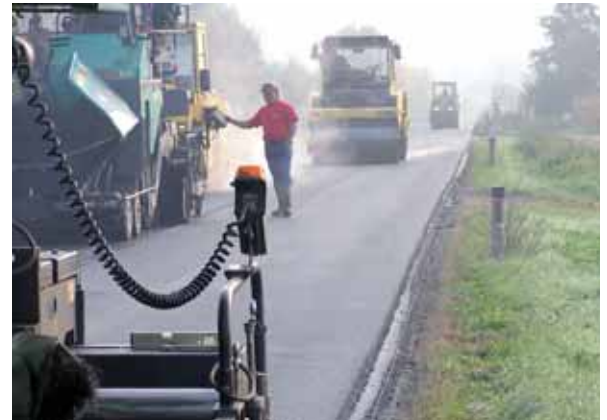
ASAplex. Installation of ASAplex modified asphalt.
