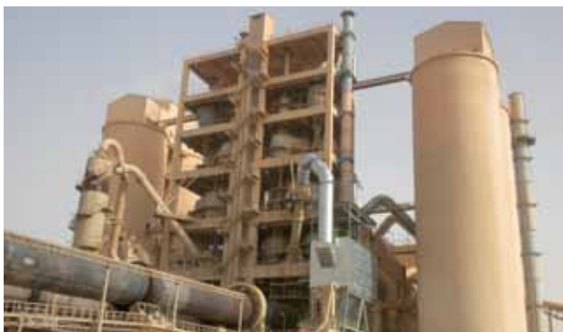
The plant in Al-Hawari (above) and Al-Fataiah (below).
