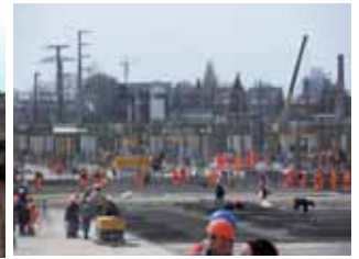
Construction work. A shopping mall in Sochi.
