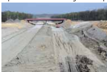
Construction site. A1 Alpine
